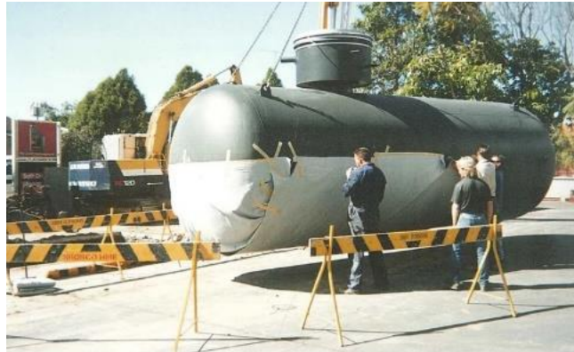
An underground LPG tank being installed at an Autogas service station
