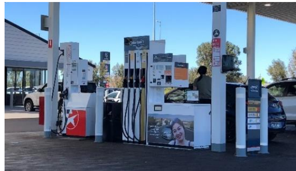
The Autogas dispenser is shown here on the left and has a delivery rate of 50 litres min
