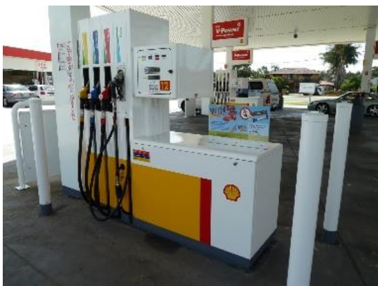
This Autogas self-serve dispenser in Australia is fully integrated with the gasoline and diesel ones
